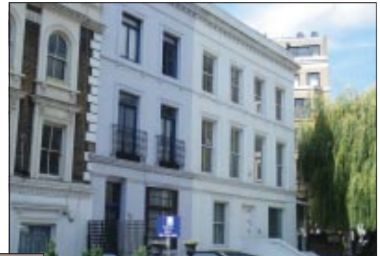
Kenway Road SW5
